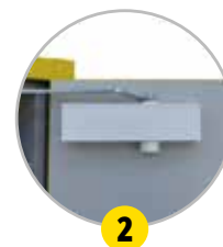
2 Self-closing door with thermo-fuse
